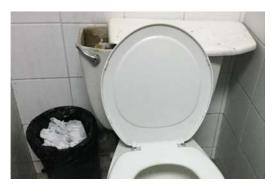
The workers reported that some of the restrooms are in a state of disrepair, including stalls without locks and broken tank lids. They reported that, for some of the toilets, the flush mechanism does not work and that the trash cans are small, and therefore overflowing, and do not have lids.
